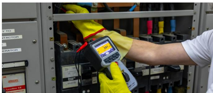
Applications requiring long test leads are not a problem for the DLRO2 as it has a dedicated long lead test to optimise the output. The long test lead function is able to provide up to 1 A of test current into 3.2 ohms resistance. This makes the DLRO2, with its optional cable reel test leads, ideal for testing wind turbine and avionic lightning protection applications.
